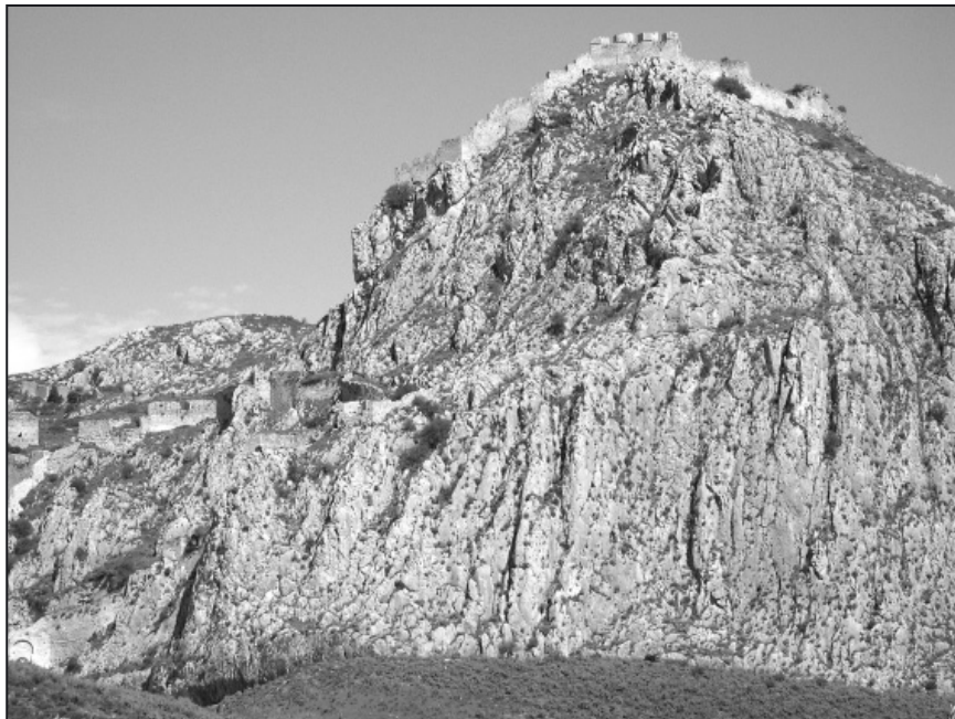
Fig. 1. The western side of Akrokorinthos Castle.
