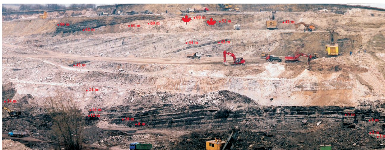
Fig. 1. Tsatsarovtsi section of the Beli Breg Lignite Basin: general view.
