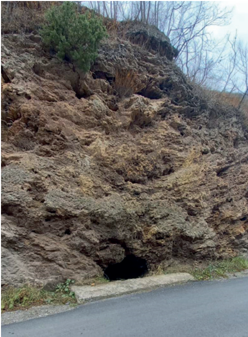
Fig. 1. Opening of the channel at the road.
